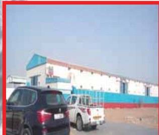
DANA STEEL - UAQ Branch
